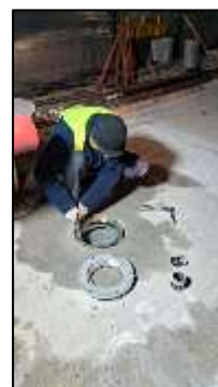
Fitting adapter rings on L-868 base
