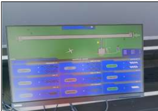
Control system installation
