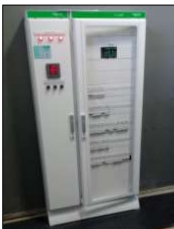
Installed Lights Board
