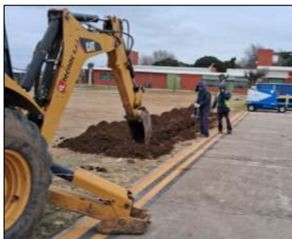
Machine trenching for primary cables
